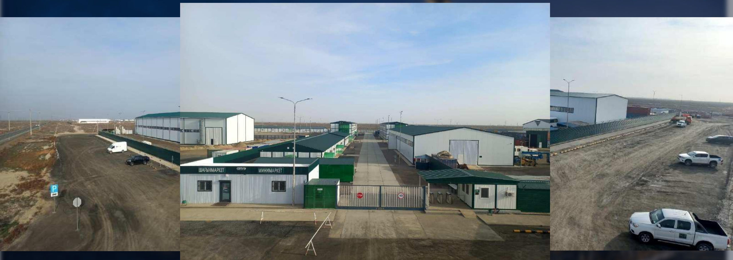
TENGIZ WORKERS' CAMP
